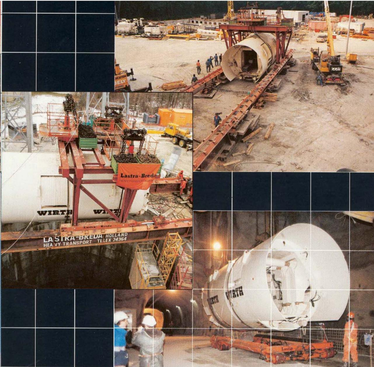
Transport and handling of 200 ton drilling equipment using gantry and self-propelled platform trailer designed by ALE Lastra.
