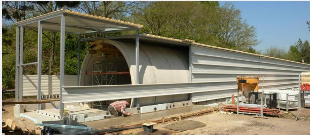
The XFEL is based on the feasibility of a single tunnel design including the support of the cryomodules from the ceiling. Installation procedures to be trained at the mock-up.
