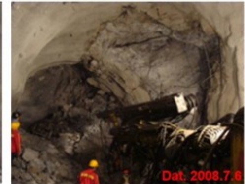
(b) Intensive rock burst of AK9+685-690m
